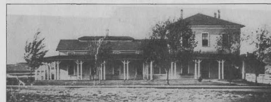
Post Hospital ca. 1880
